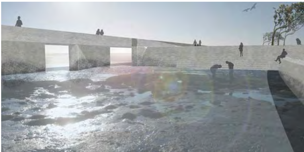
Figure 24: the proposed wave breaker underneath the coastal promenade absorbs the power of the tide, but allows the water to filter through at a controlled pace to allow the mudflats to thrive
